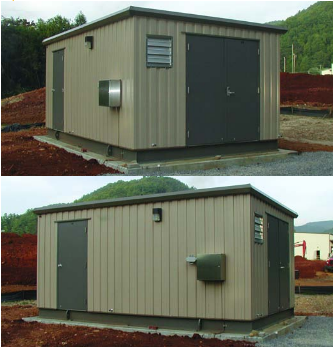
The Erwin pump station is mounted with interconnecting piping and wiring inside a pre-fabricated building that includes all utilities, lighting, environmental controls, ventilation, and plumbing.
