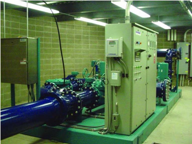
**In-line VFDs are some of the keys to this successful upgrade that improved pressure and flow reliability in the pre-fab booster station.**
