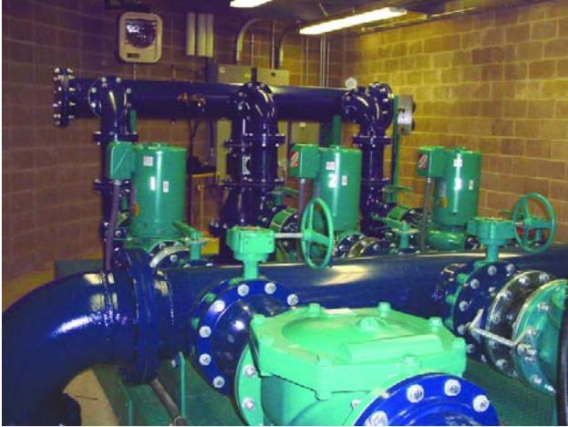
To provide reliable 24/7 storage for residential service at both higher and lower elevations, as well as industrial fire suppression up to 2,400-gpm @ 72-psi for three hours, the engineer specified a 3-pump booster station to be installed within base of new, additional storage tank. The pumps connect to a discharge manifold.
