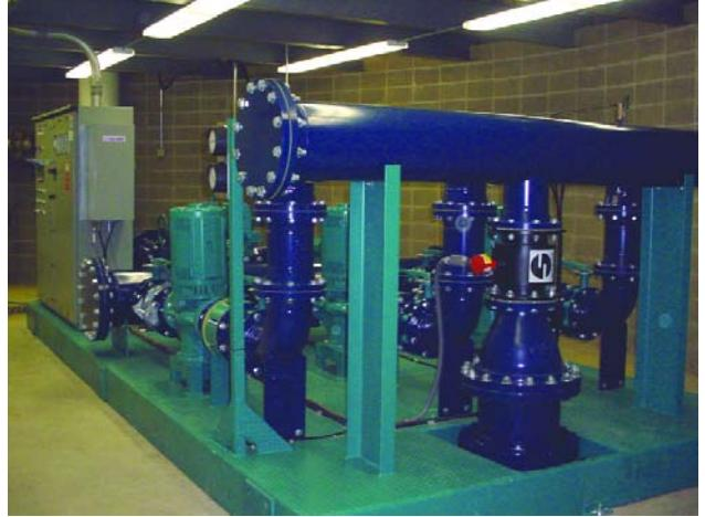
A custom "bell" adapter provides connection from the booster station to the system's discharge line. The system serves about 7,600 metered customers, 85 percent being residential and the rest business, commercial, and industrial. Peak daily consumption is 2.8-mgd, with the average at 1.6-mgd.
