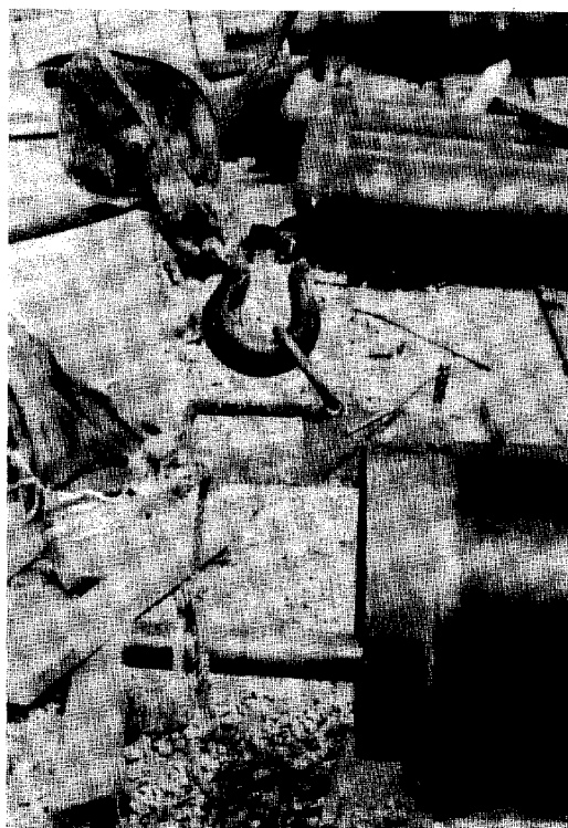
Fig. 7-5. Shaft Section Fastened To Lower End Of Column Section With Rope And Clamp. Dragline Hooked Onto Same Clamp.
