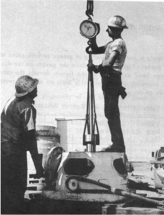
Figure 18. Tensioning the tube nut.
